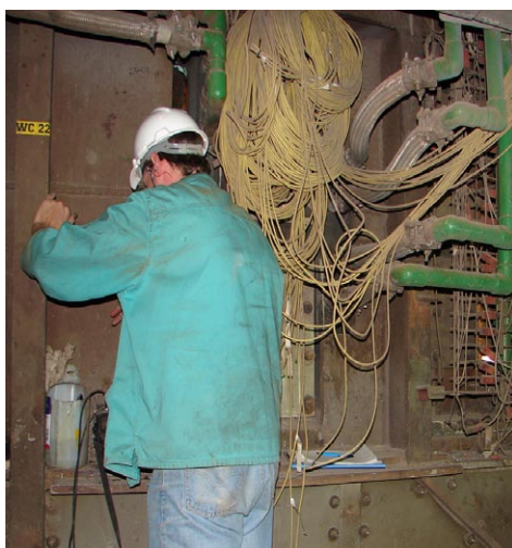
Copper cooler field inspection
